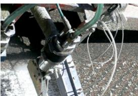
Cold plastics are reactive two- or multicomponent systems formulated with DEGAROUTE\* binders based on methyl methacrylate (MMA) and brought to polymerization by the addition of the curing component (hardener) immediately before application. The system cures chemically after a certain lapse of time (pot life), when the volatile resin components are chemically bound in the resulting inert duroplastic polymer. Thus application can be considered to be almost **free from VOC emission.**
